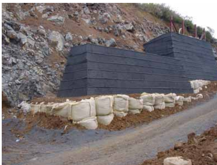
堤防型補強土防護壁
